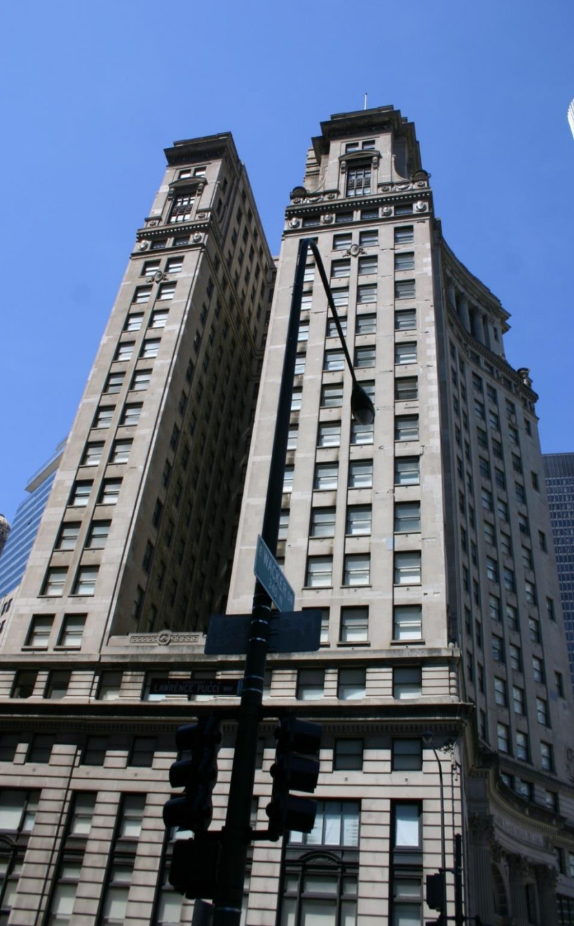
Chicago, 1837: London Guarantee Bldg (1923, 22 fl, 96 m), on North Michigan Avenue.
